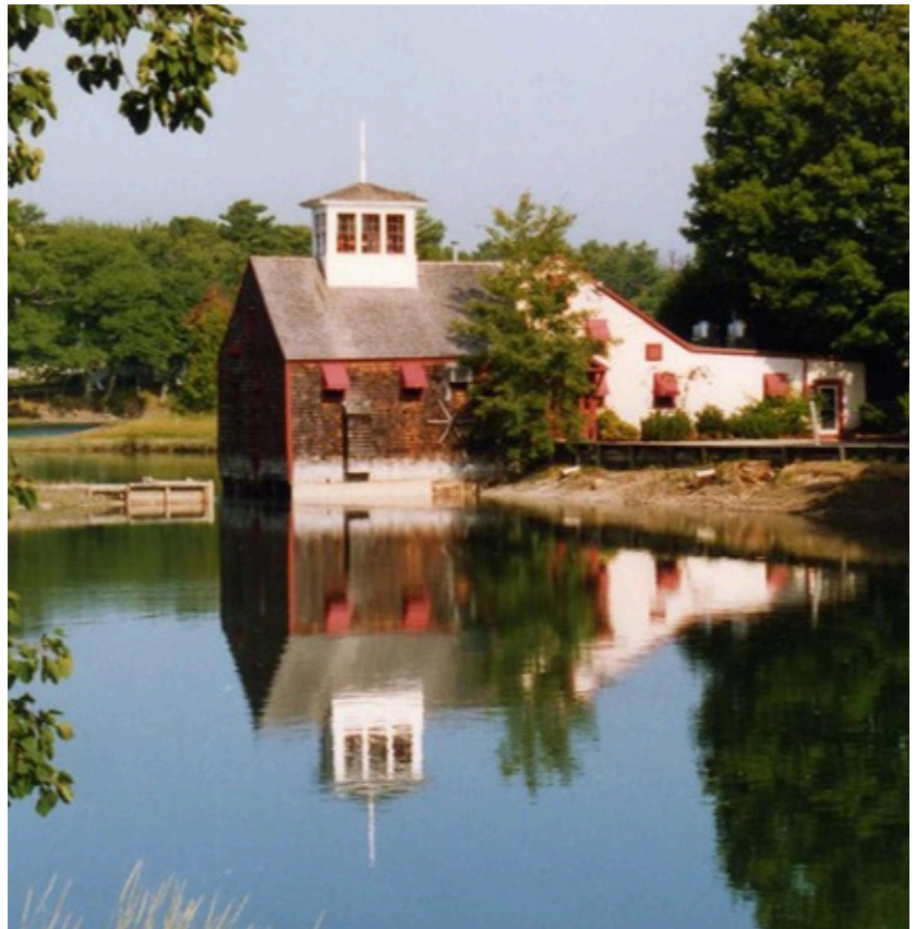
The historic Grist Mill, which stood on this site since 1749, was lost to fire in 1994.
